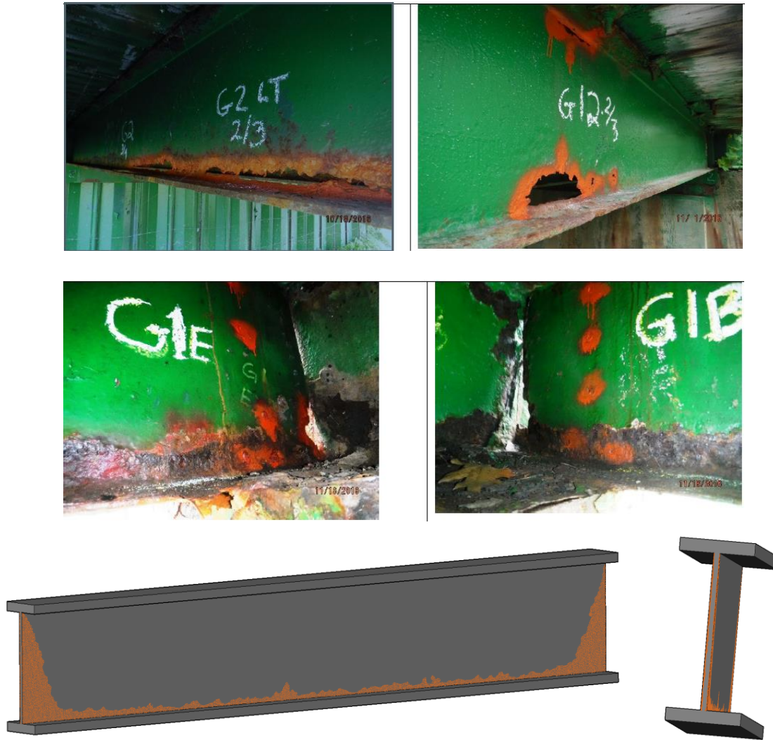
Figure 1: Typical Steel Girder Corrosion at Web and Flange
